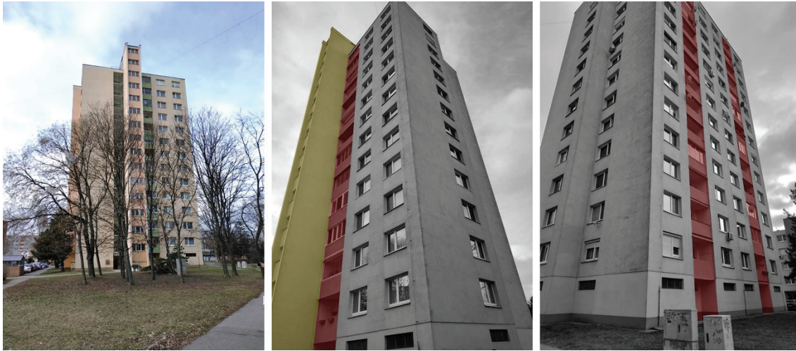
Fig. 1 Existing status of apartment building. The red space indicates the space which is the subject of alternative positions to the heated volume. The staircase buffer area is indicated in yellow.
